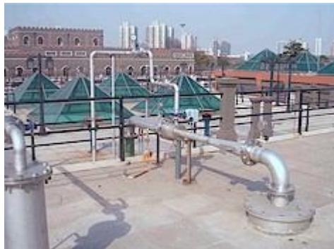
Furthermore Degrémont Technologies-Ozonia has delivered two thermal VOD, the diffusing systems for pre- and post-ozonation, the closed cooling water circuit and all necessary instruments and valves. The drinking water plant is located in Shanghai and has a capacity of 375'000m<sup>3</sup> / day.
