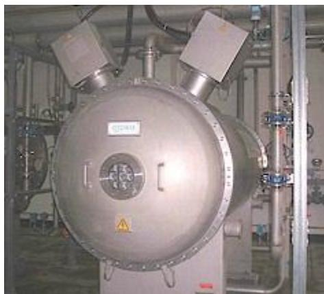
Exhaust gases from processes where ozone has been used invariably contain residual amounts of un-reacted ozone. Before this exhaust can be vented to atmosphere it is necessary to decompose the traces of ozone. In most countries it is forbidden to exhaust even low concentrations to atmosphere. There are various methods available to treat vent gas.
