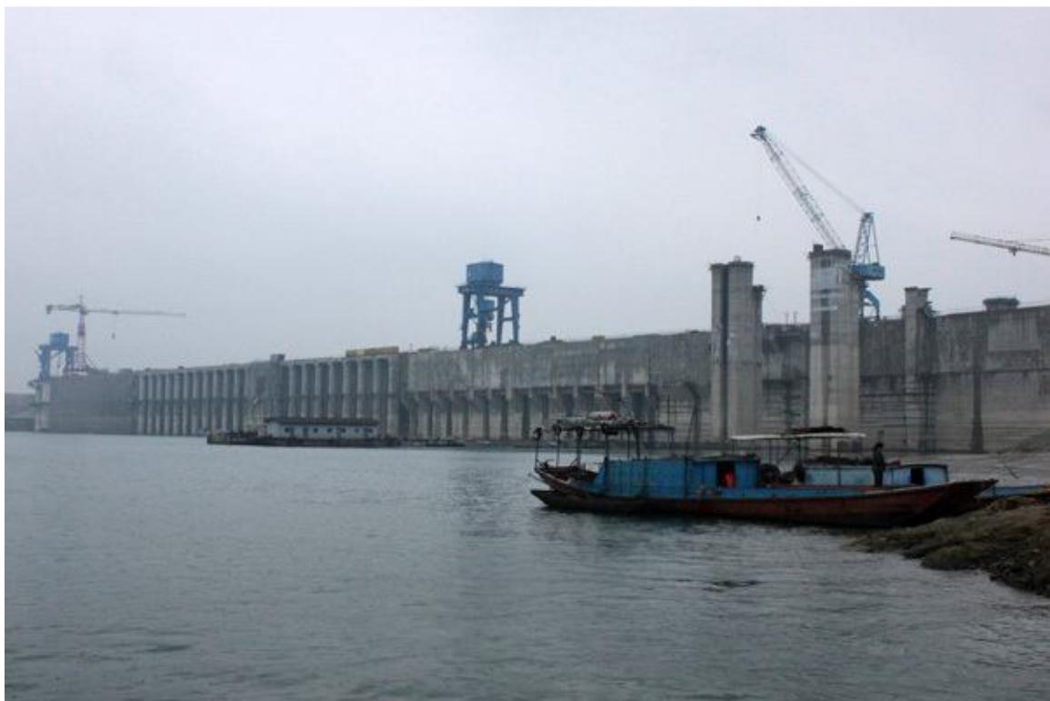
The Danjiangkou Reservoir is being constructed, and now the height of the reservoir has reached 176.6 meters from 152 meters. [China.org.cn]
